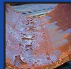
ICDA 307 Pipelines 2,725 KM
