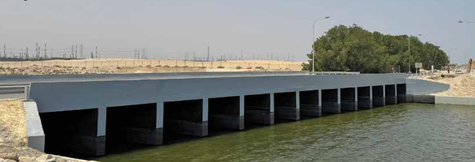
Recently completed Concrete Cathodic Protection for Box culvert in Saudi Arabia
