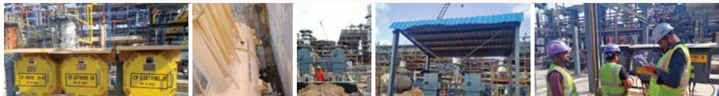
BSS Technologies has successfully completed Cathodic Protection System for Underground Vessels DCU WITH UNSATURATED LPG TREATING UNIT, Diesel Hydro Treating Unit (DHDT) & Hydrogen Generation Unit (HGU) & VGO Project at HPCL RAJASTHN REFINERY LIMITED.
