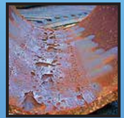
ICDA 335 Pipelines 3,010 km
