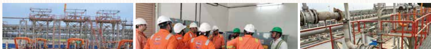
BSS Technologies Successfully completed CP system for LPG Mounded Bullets at ACRYLIC / OXO ALCOHOL PROJECT AT GUJARAT REFINERY, DUMAD COMPLEX. The job included Detailed Design, Supply, installation, commissioning & interference.
